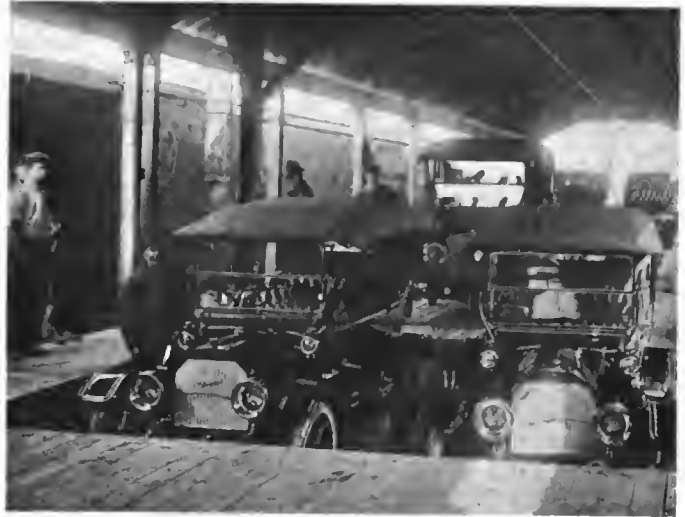
The Studebaker shipping organization, like that of nearly every other Detroit automobile plant, cultivates efficiency. The illustration shows an hydraulic elevator lifting cars from the factory yard to the loading level. Car can be brought to the platform regardless of the position of trains on the sidings. The shipping equipment of the company represents an investment of $60,000. The switch tracks back of the plants are 20 feet above the level of the factory and the new loading platform is a massive shelf as long as two city blocks, with railroad sidings
